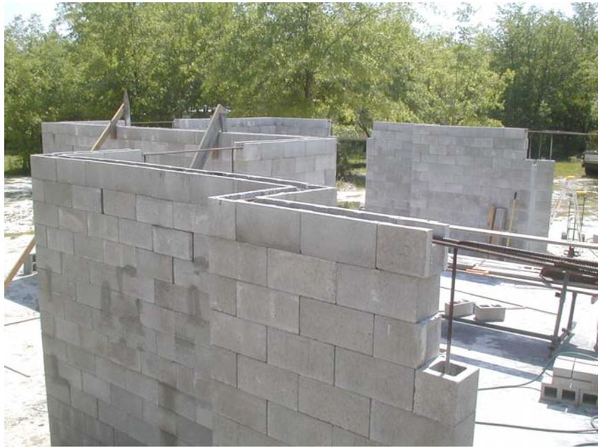
**Figure 39. Corner blocks and linear half blocks.**
